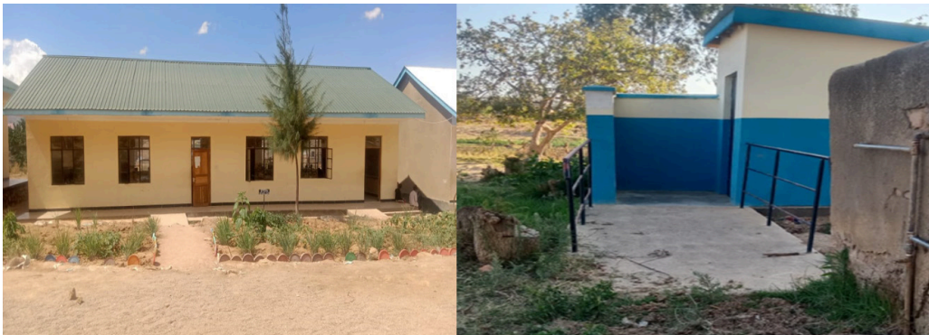
Picture 7: A renovated classroom at Kihesa Secondary School (left) and a toilet for children with disabilities constructed at Mgama Primary School (right) in Iringa
