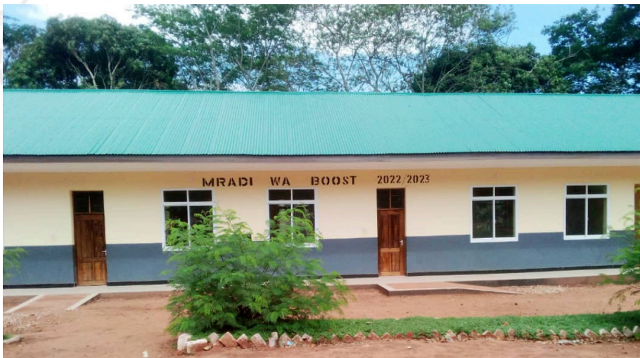
Picture 8: New classrooms at Kiheba Primary School in Kigoma
