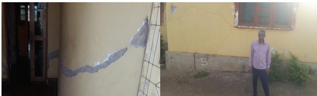
*Picture 74: Cracks at the house of one of the villagers of Nyamalambo reportedly caused by GGM mining operations*
