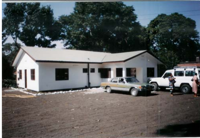
A newly-renovated LHRC Arusha Office
